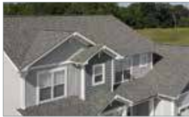
Roofing and Ventilation
