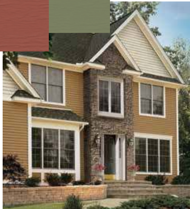
Siding: Monogram Double 4" Clapboard in mountain cedar with Cedar Impressions Triple 5" Straight Edge Perfection Shingles in sandstone beige.
